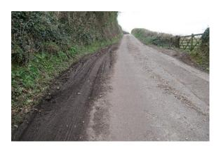
During the period of closure vehicles were required to move off the made-up surface of Water Hill onto the soft verge which quickly became torn up, having coincided with a period of heavy rain. This became a safety issue due to the steepness of the hill and slipperiness of the 'off road conditions' as vehicles tried to pass one another.
